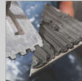
Cement Laying On Tile
