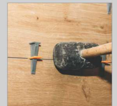
Remove Wedges Ones It Dry
