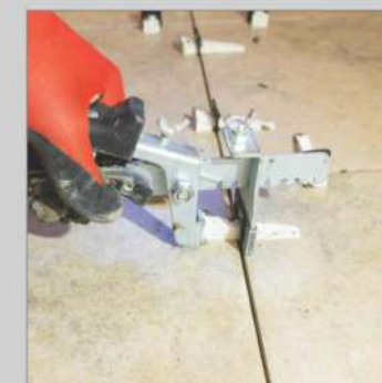
Levelling Wedges
