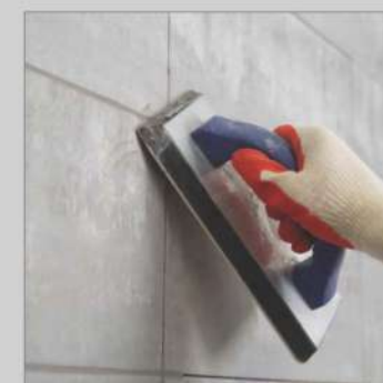
Joint Grouting
