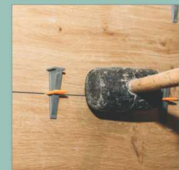
Remove Wedges Ones It Dry
