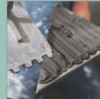
Cement Laying On Tile
