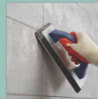
Joint Grouting
