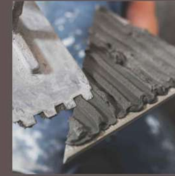
Cement Laying On Tile
