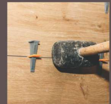
Remove Wedges Once It Dry
