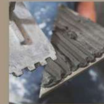
Cement Laying On Tile
